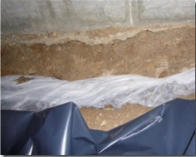
The trenches are filled with rocks and wrapped with a special cloth, which allows the water to be collected and sent down stream. These trenches then feed into two catch buckets at the centers of each end of the house. The buckets contain a 1/2 hp pump for pumping the water out. They also have a battery-operated water alarm connected to it, in case of failure and overflow.
